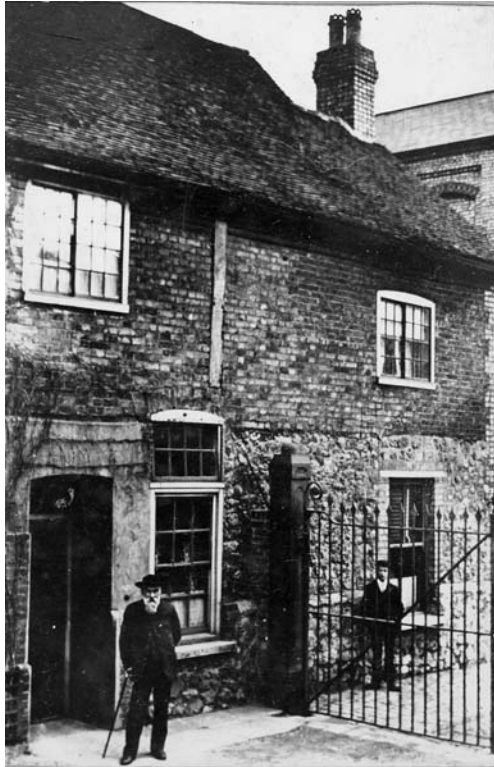
The first Independent Chapel in Mill Street
